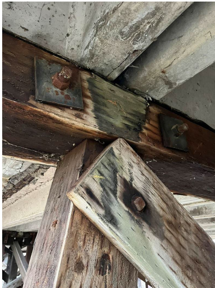
Figure 2-8: a) and b) Bent-4 Cap shows degradation.
