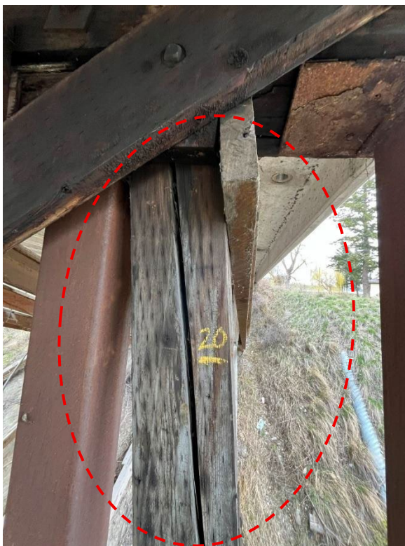
Figure 2-15: Pile cap bent 3 decayed and crushing over the timber columns.
