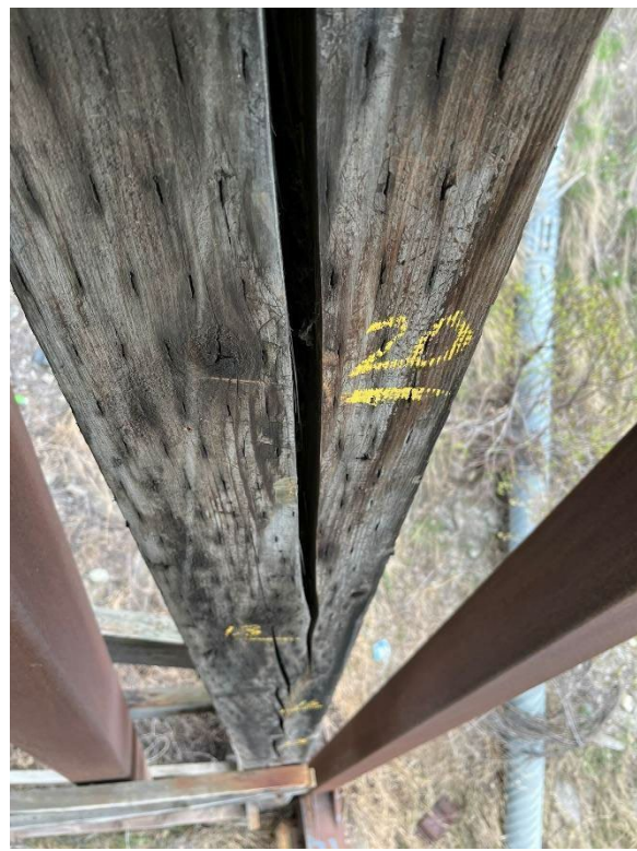
Figure 2-15: Pile cap bent 3 decayed and crushing over the timber columns.
