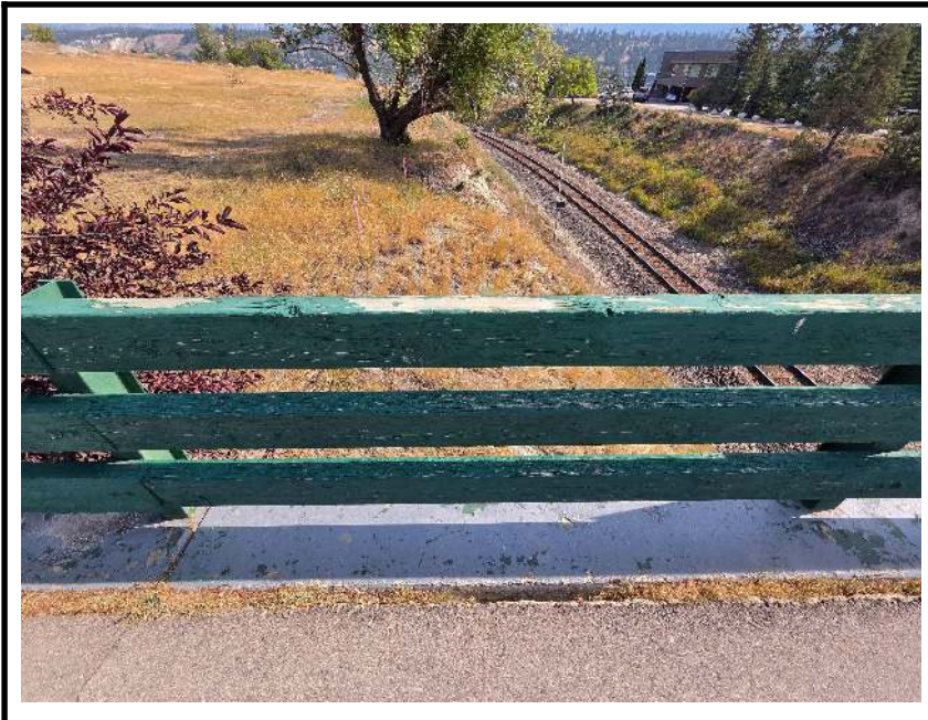
Photo 2: Green paint sampled in the Project Area (Handrail) contains 2460 \mu\text{g/g} of lead
