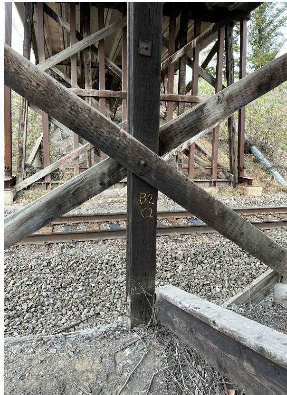
Figure 2-10: Bent 2, column 2 - detailed zoom view.
