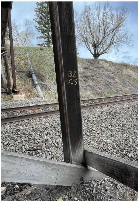
Figure 2-11: Bent 2 Column 4 large shrinkage check.
