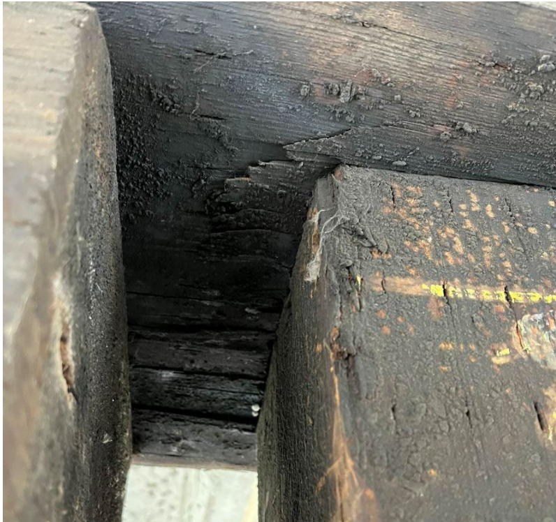
Figure 2-15: Pile cap bent 3 decayed and crushing over the timber columns.
