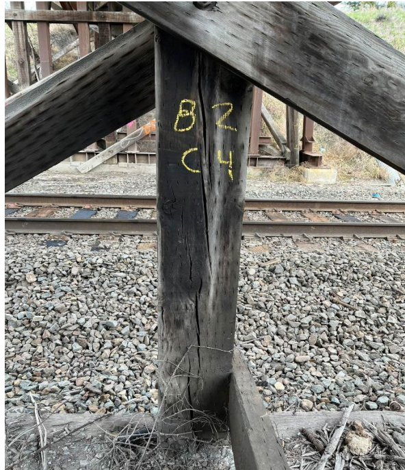
Figure 2-11: Bent 2 Column 4 large shrinkage check.
