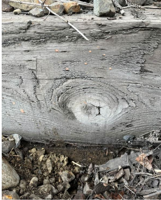
Figure 2-13: Bent 2 bottom sill founded on concrete footing.
