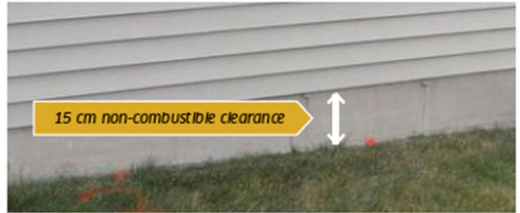
HAZARD FACTOR 7: GROUND TO SIDING CLEARANCE
